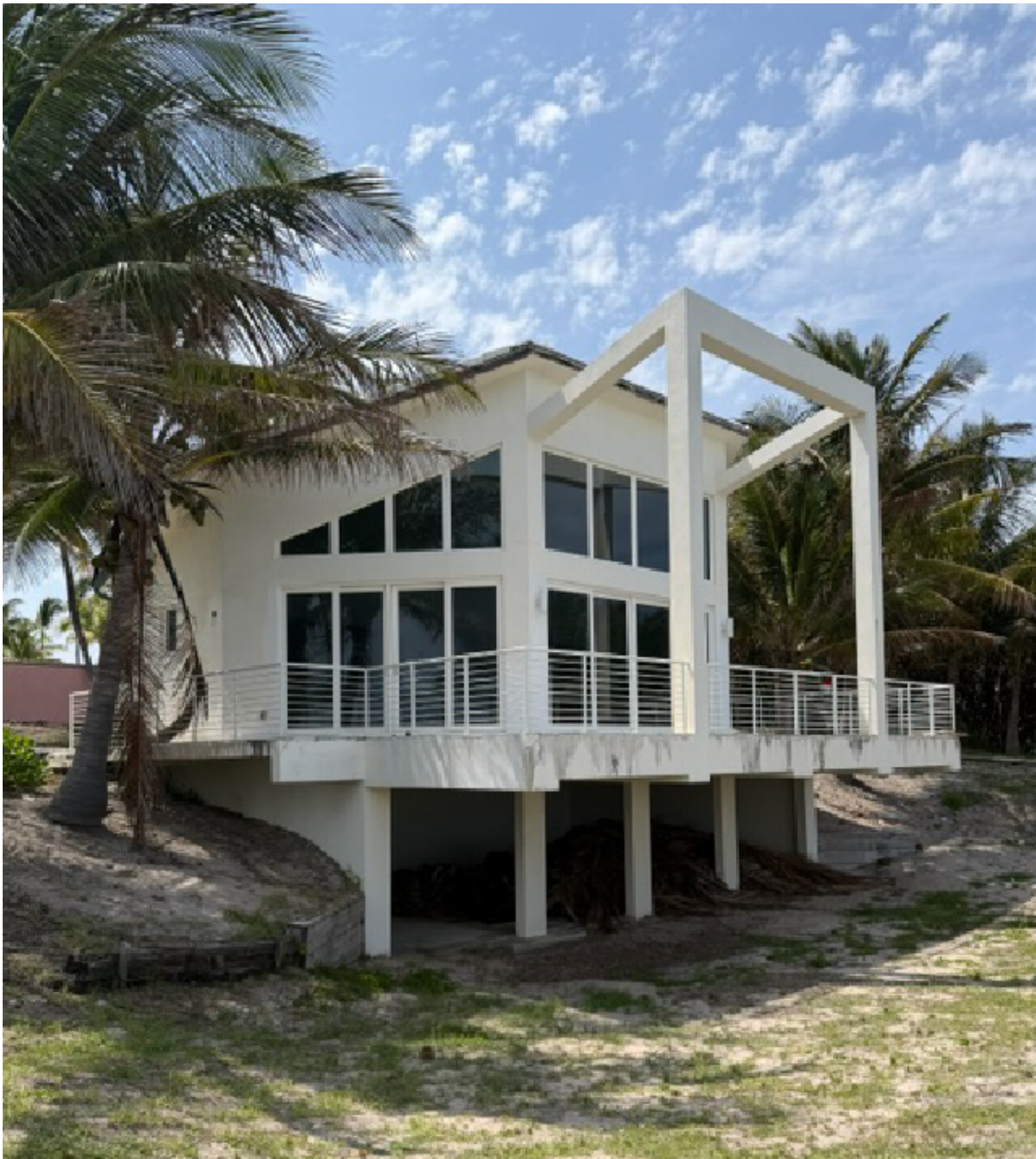
VIEW FROM THE NORTHEAST
