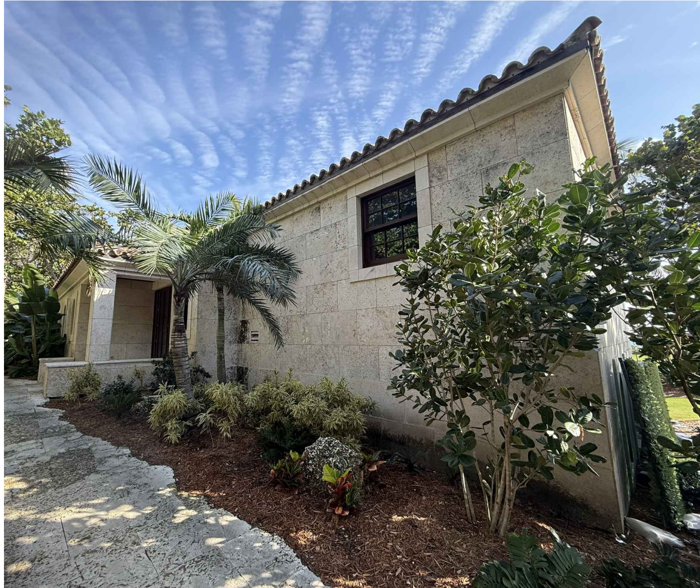
EXISTING VIEW TAKEN FROM SOUTHWEST
