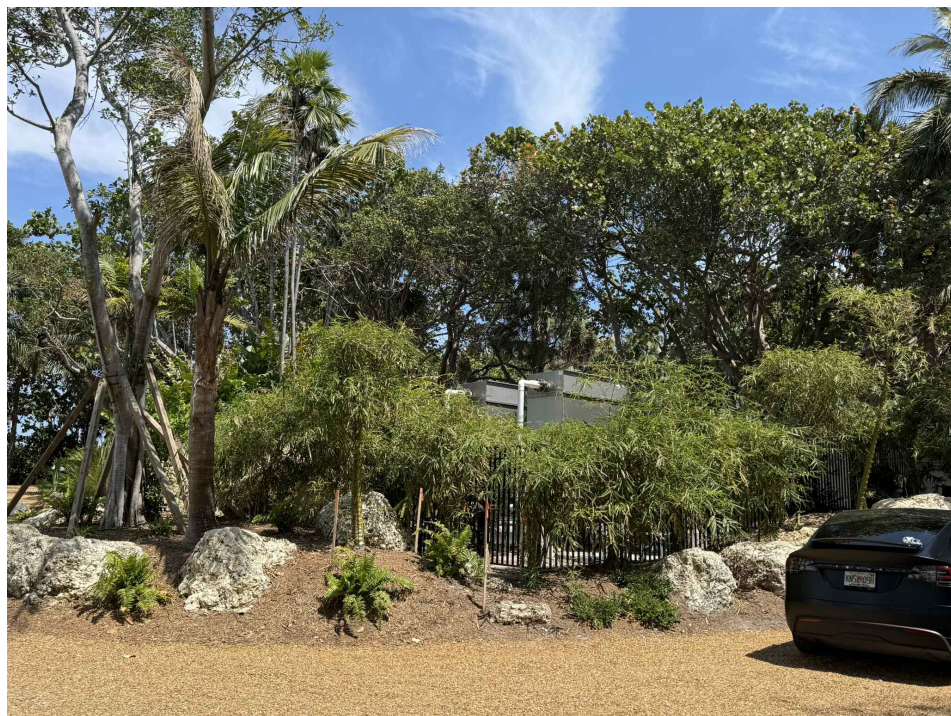
EXISTING COOLING TOWER AND ENCLOSURE - VIEW C
